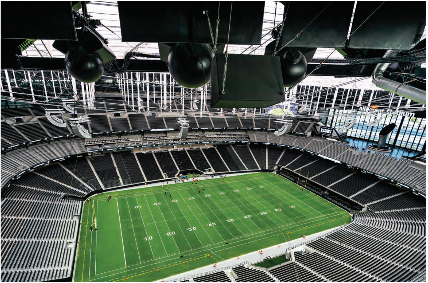
MATSING LENS ANTENNAS POINT DOWN FROM THE ROOF'S OUTER RING. CREDIT: MATT AGUIRRE/LAS VEGAS RAIDERS
