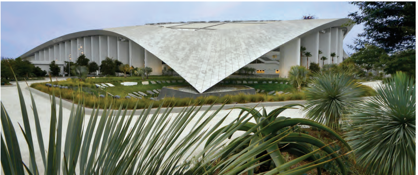
CLOCKWISE FROM TOP LEFT: TEAMS ON THE FIELD AT THE CHARGERS' FIRST HOME GAME (CREDIT: TY NOWELL/LOS ANGELES CHARGERS); THE STADIUM DURING CONSTRUCTION; AN OUTSIDE STADIUM VIEW.
