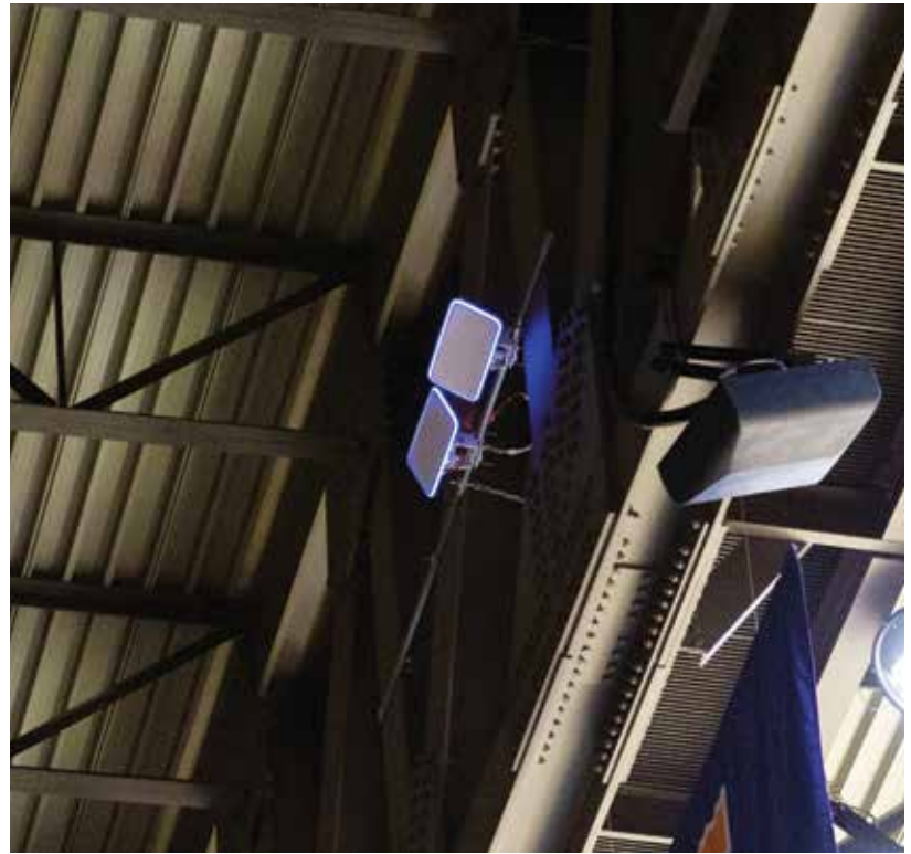
FROM LEFT: WI-FI ANTENNAS ARE INTERSPERSED WITH OTHER RAFTERS GEAR; RIGHT, TWO APS TILTED AT DIFFERENT ANGLES (NEAR A DAS ANTENNA)
