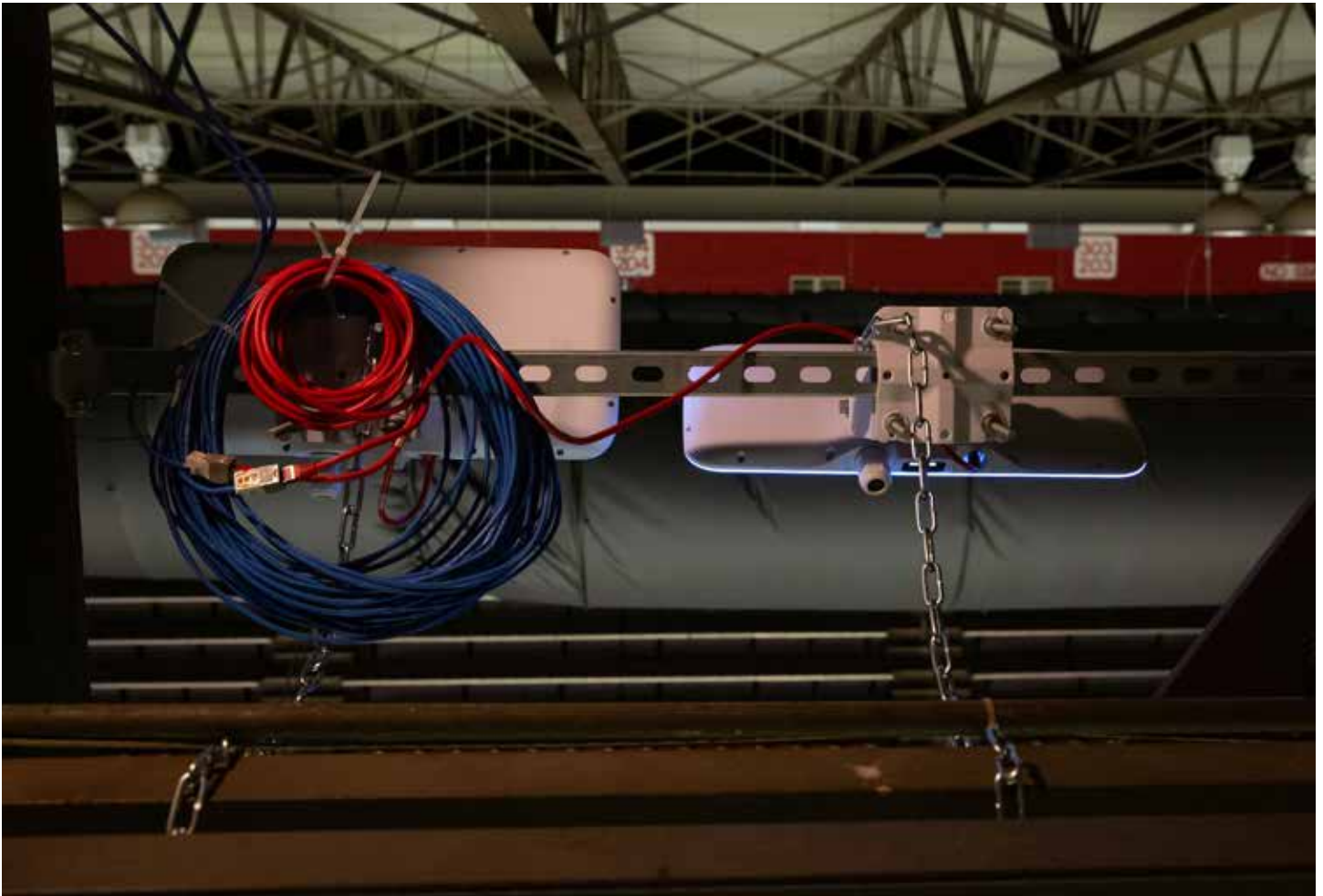
A TOP-DOWN LOOK AT THE ANTENNA MOUNTING SOLUTION.
