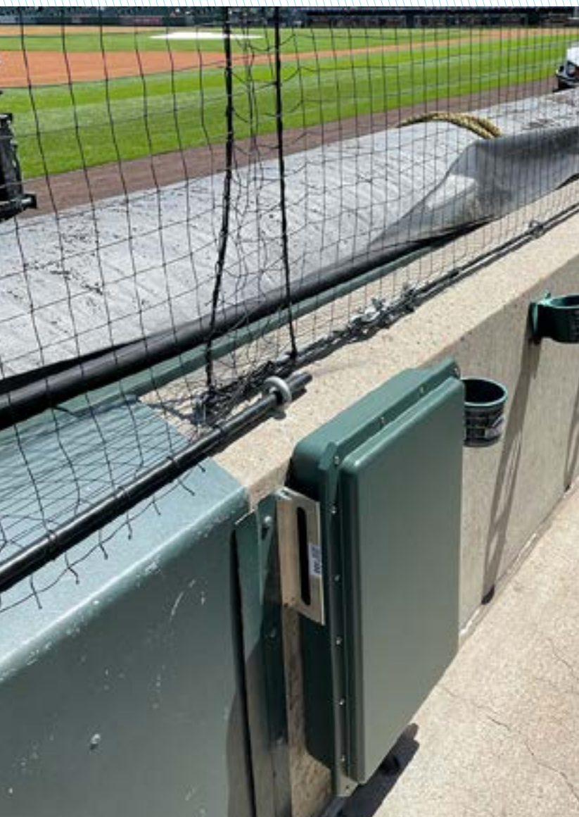
A slimmer 'coffin' enclosure points back from the field wall to lower-bowl seats.
